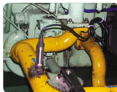
Oil Humidity Sensor Installed
