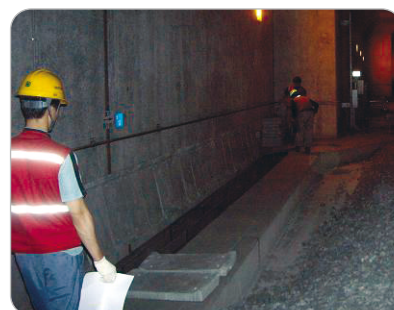
RTU Communication Cabling Work
