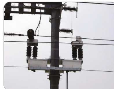
Open/Close Switch Installed
